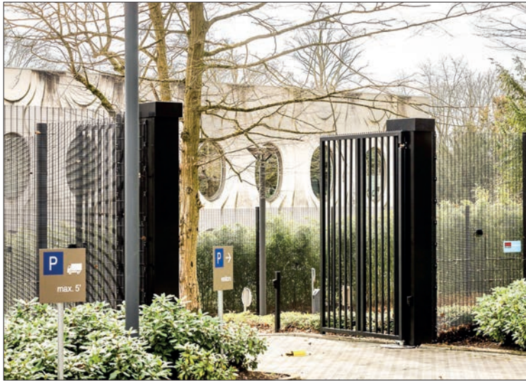
The headquarters of SWIFT, Society for Worldwide Interbank Financial Telecommunication, in La Hulpe, Belgium near Brussels. PHOTO: BELGA/AFP
