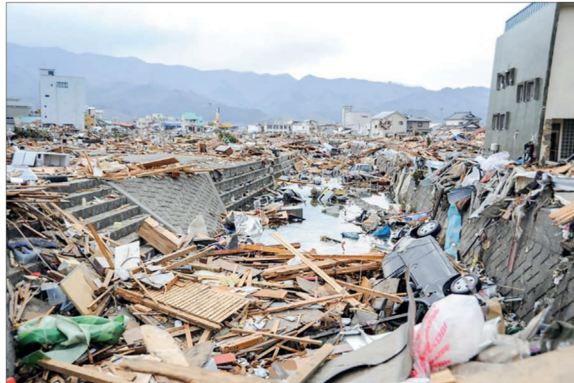
Damage of Tsunami caused by Great East Japan Earthquake in 2011
