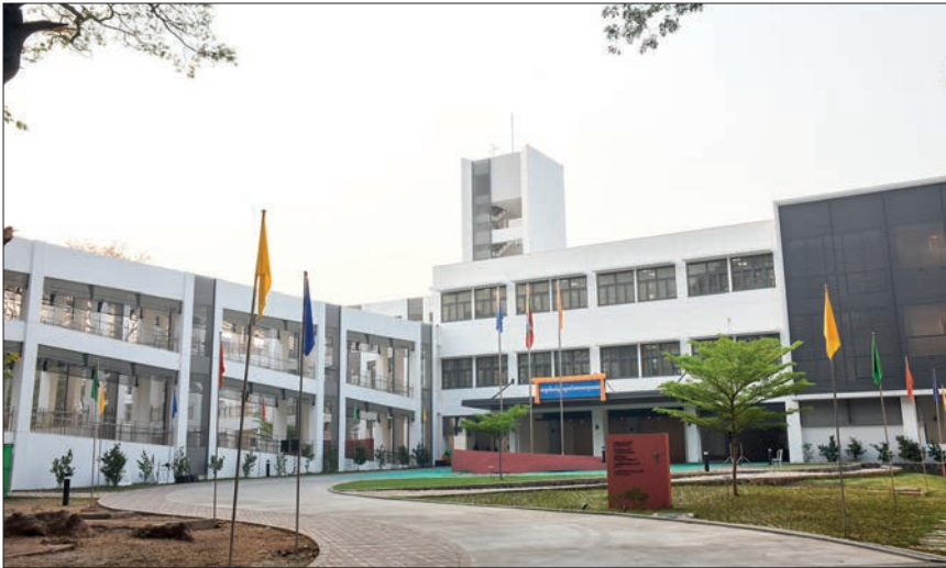
The outside and inside view of the new maternity and newborn babies ward.
