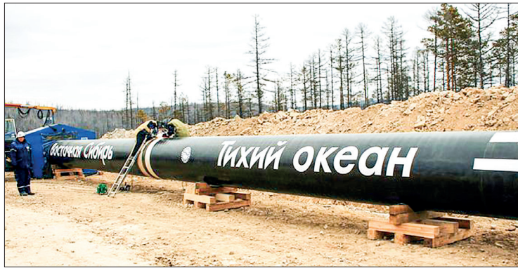
Workers weld a juncture for a Russian oil pipeline in Siberia in this file photo. PHOTO: AFP
