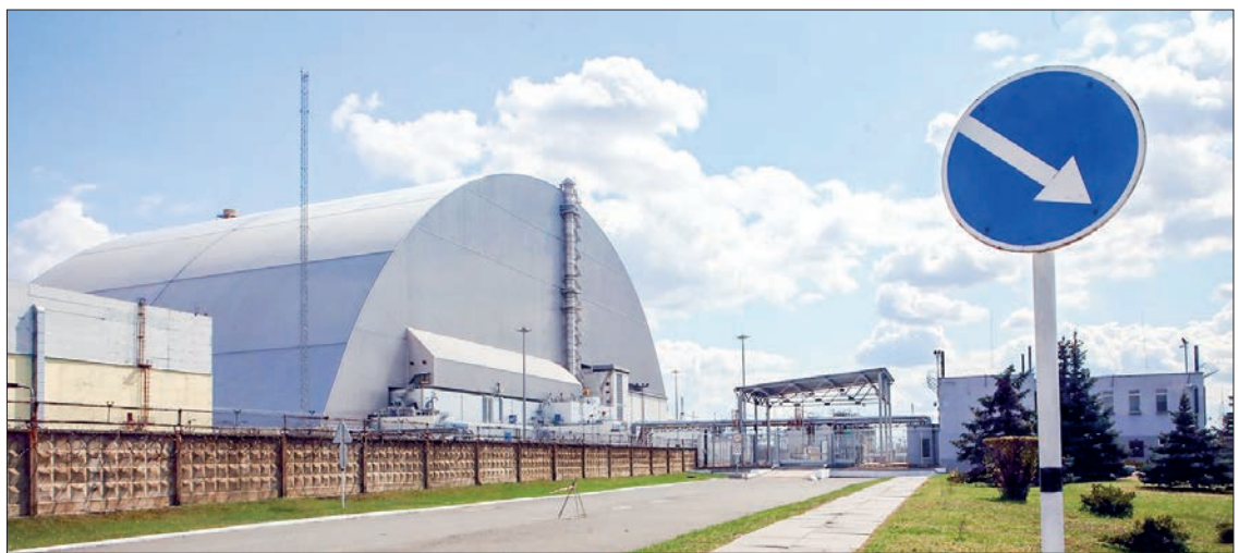
The New Safe Confinement seals off the Object Shelter, also known as the Sarcophagus, a temporary structure built in 1986 over the debris of the 4 th reactor of the Chernobyl Nuclear Power Plant, Kyiv Region, northern Ukraine. PHOTO: FUTURE PUBLISHING/XINHUA
