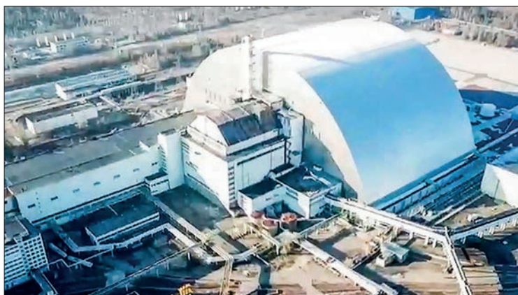
The defunct nuclear power plant still uses electricity to keep spent fuel at manageable, safe temperatures. PHOTO: RUSSIAN DEFENCE MINISTRY/XINHUA
