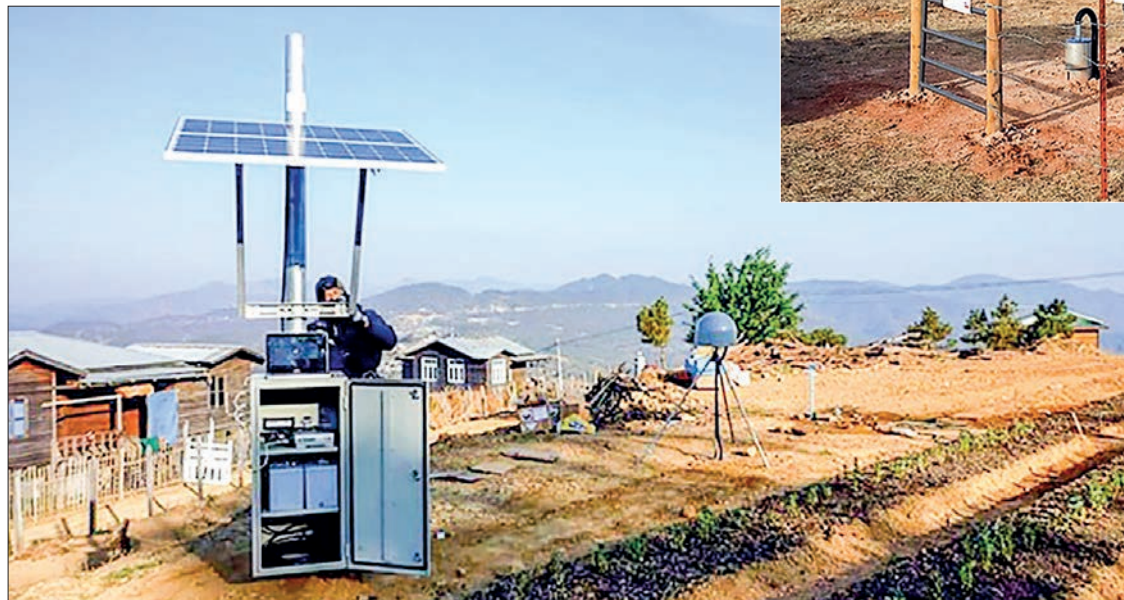
The photos show the installation of seismometers and GPS devices in Yangon Region.
