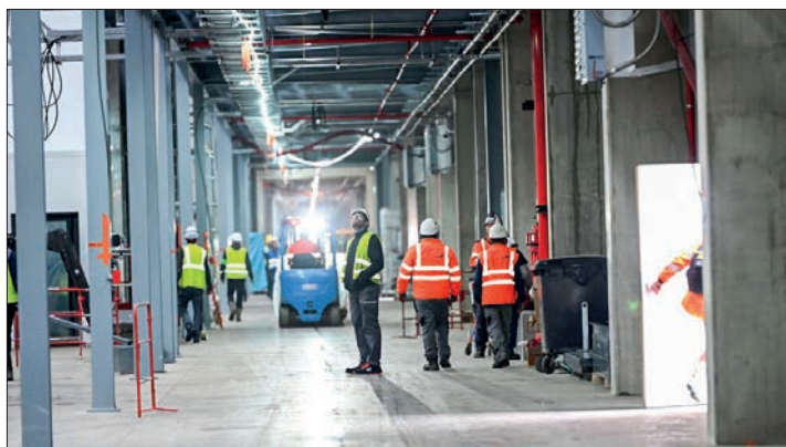
This photograph taken on 9 May 2023 shows workers at the site of the newly constructed Billy-Berclau Gigafactory ACC battery factory, in Billy-Berclau, northern France. PHOTO: FRANCOIS LO PRESTI, AFP/FILE
