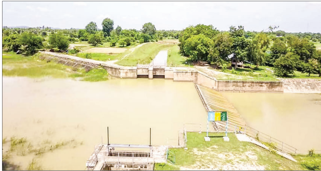
The view of Chaungmagyi Dam.
