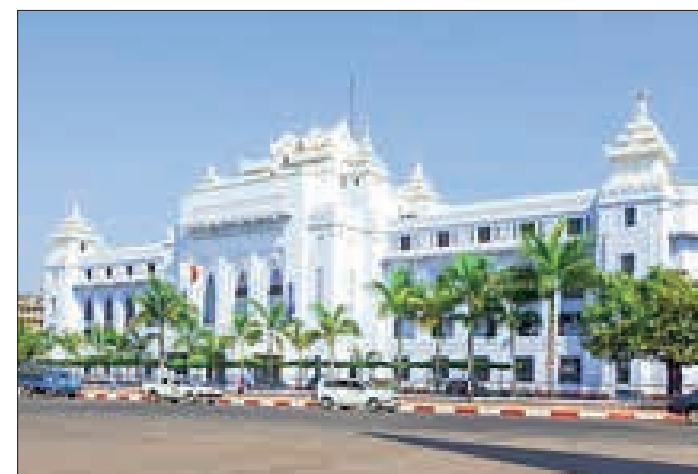
The office building of the Yangon City Development Committee.
