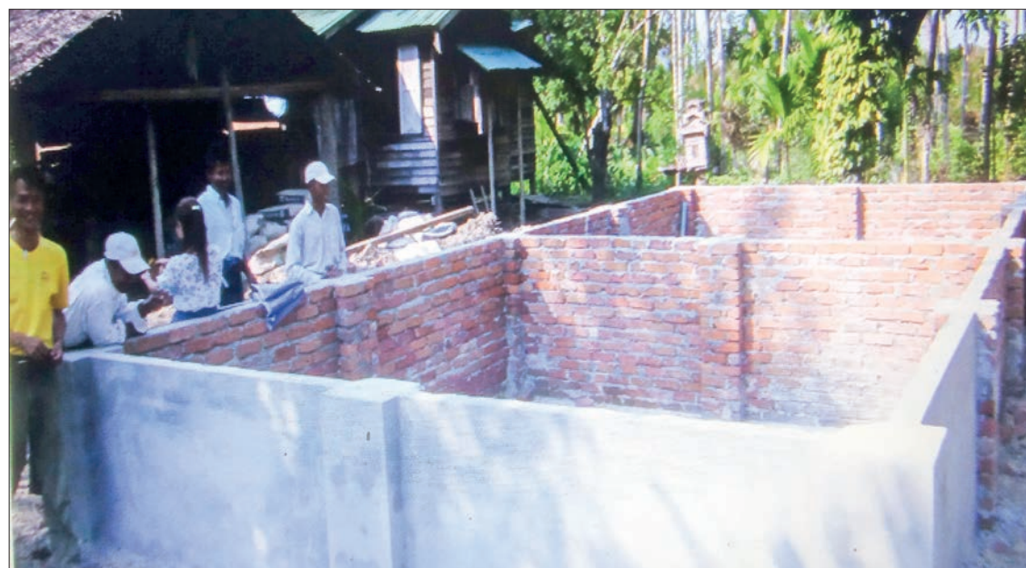
For eel farming on a manageable scale, two (2x1x1 metres) ponds must be adjacent. The surface area of the two ponds is four square metres. Mud must be put into half of the lake (ten centimetres).
