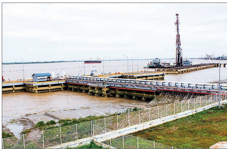
The photo shows the Thilawa Port Terminal where fuel oil is unloaded.
