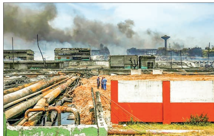
Sixteen firefighters were killed and 17 others hospitalized due to a massive fire in Matanzas, on Cuba's northern coast. PHOTOL AFP
