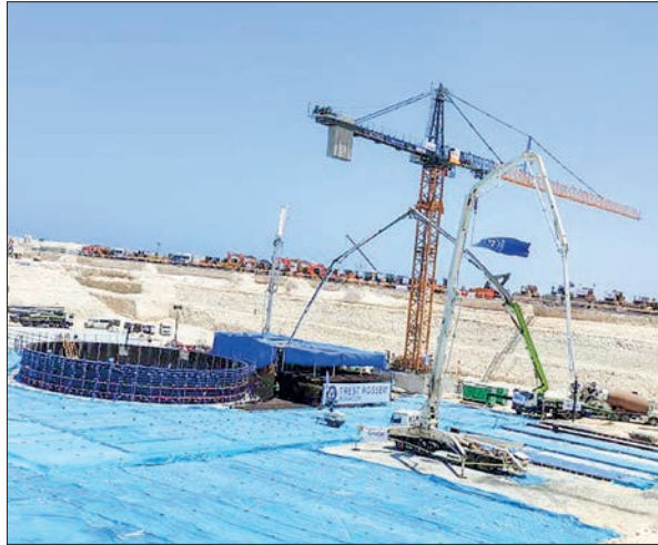
Under the deal worth three trillion won ($2.25 billion), a South Korean company will reportedly supply the equipment and a Russian firm will be in charge of constructing the reactors at Egypt's first nuclear power plant in the northern city of El Dabaa. The first concrete is poured for unit 1 of the El Dabaa plant. PHOTO: THE NUCLEAR POWER PLANTS AUTHORITY (NPPA)
