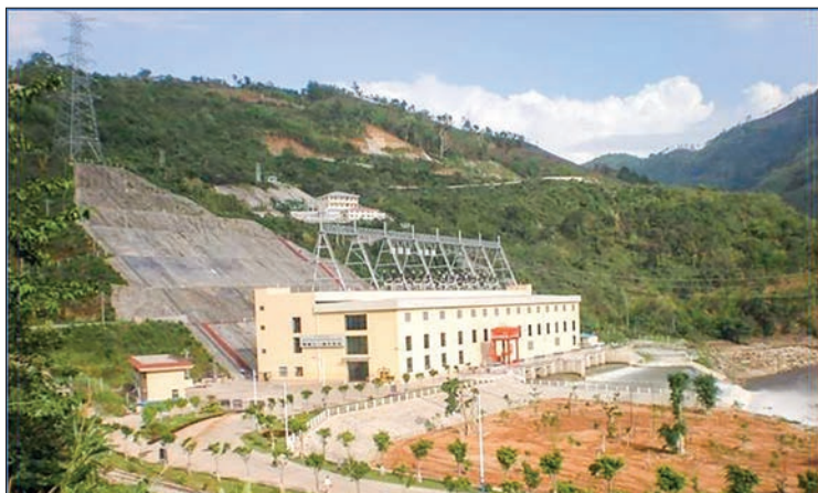
The Shweli Power Plant No 1 in Namhkam Township, Shan State.
