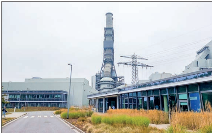
Russia's curtailing of gas exports to Germany in the wake of the Ukraine war has forced Berlin to make the radical decision to restart coal power stations, at least temporarily. PHOTO: AFP
