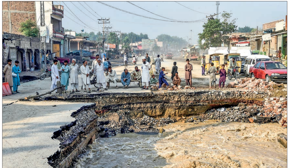
Residents gather beside a road damaged by flood waters following heavy monsoon rains in Charsadda district of Khyber Pakhtunkhwa on 29 August 2022. PHOTO: AFP
