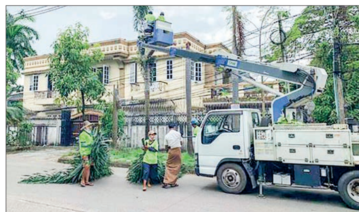
YESC was removing trees and branches touching power cables in Hline Township of Yangon Region in 2021.
