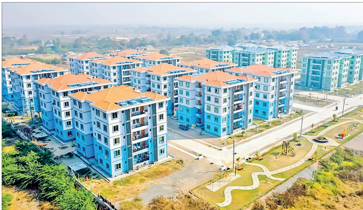
A construction status of the public rental housing project is seen in Mandalay.
