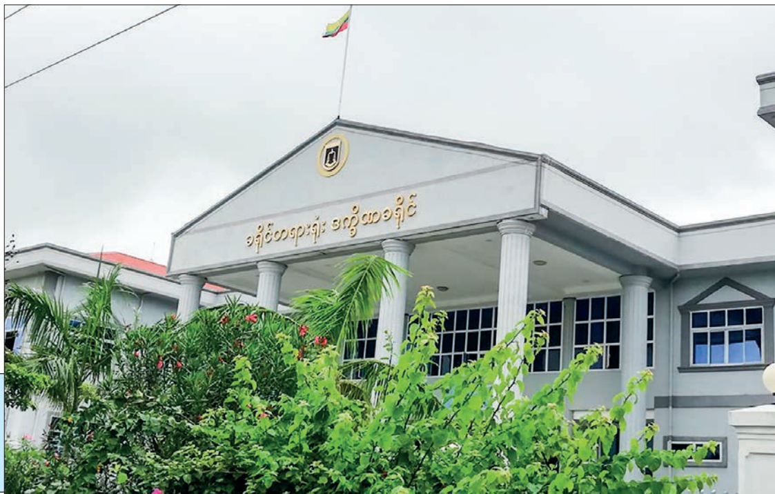
Photo shows Dekkhina District Court in Nay Pyi Taw.
