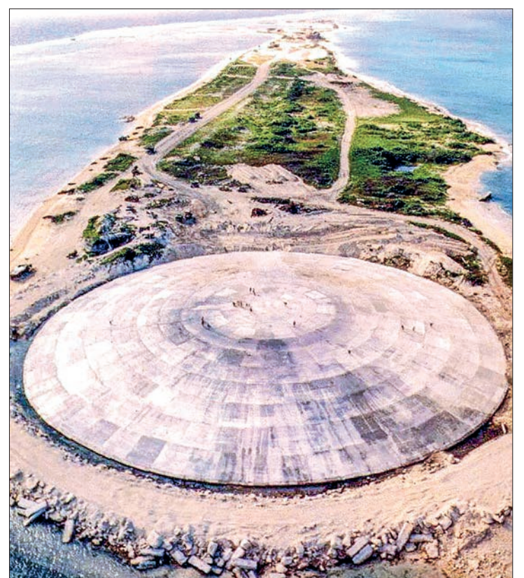
The huge dome built over the top of a crater left by one of the 43 nuclear tests over Runit Island in Enewetak in the Marshall Islands. PHOTO: AFP
