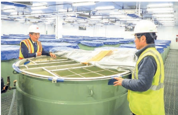
Asahi Shuzo Co CEO Kazuhiro Sakurai (L) examines one of the tanks to be used to brew sake at his company's new plant in Hyde Park, New York, on 19 Oct 2022.
