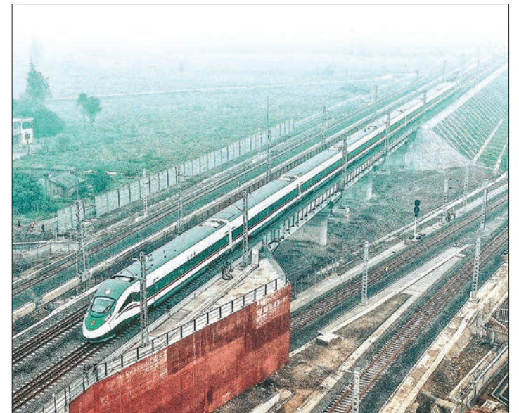
A Fuxing bullet train travels by Emeishan city in Sichuan province on Friday on the new Chengdu-Kunming rail line. PHOTO: HE HAIYANG/FOR CHINA DAILY
