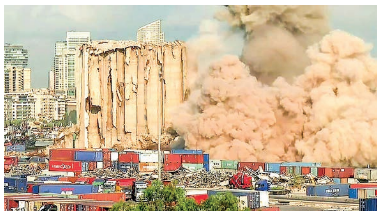
Smoke plume rising after the new collapse of the northern section of the grain silos at the port of Lebanon's capital Beirut, which were previously partly destroyed by the 2020 port explosion. PHOTO: DYLAN COLLINS/AFPTV/AFP
