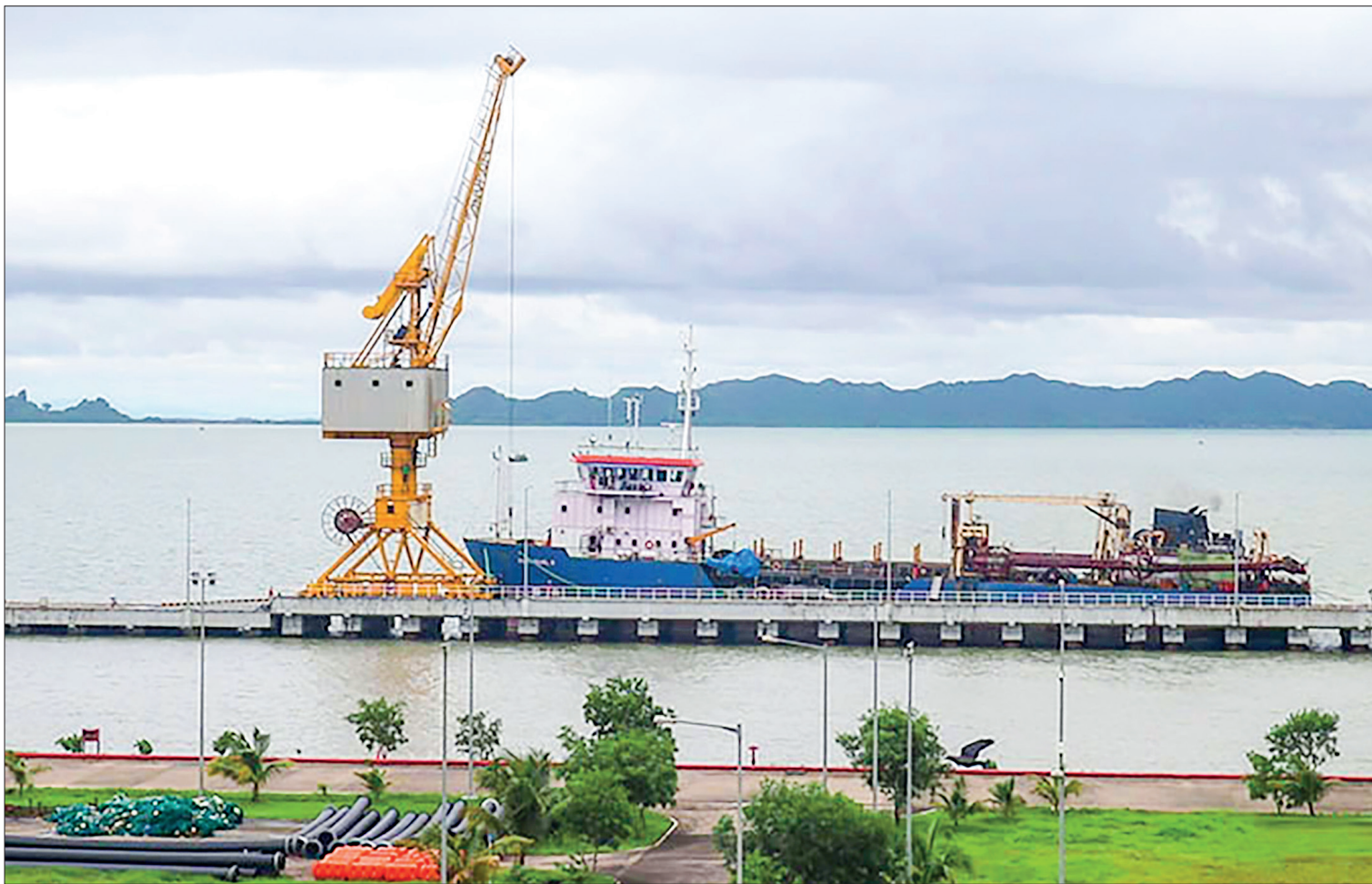
General view of the Sittway Port construction site.
