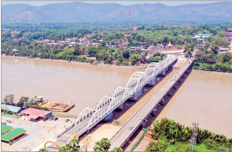
An aerial view of already-opened Kamyawkin Bridge.
