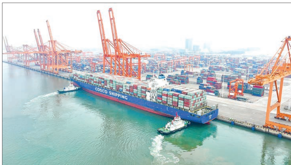
Photo taken on 2 March 2022 shows a container terminal of Qinzhou Port in south China's Guangxi Zhuang Autonomous Region. PHOTO: XINHUA
