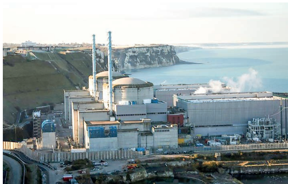
The crack was discovered in a cooling pipe at a reactor on the Channel coast. PHOTO: AFP/FILE
