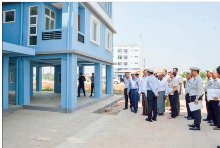
Yangon Mayor U Bo Htay views round the Yangon Region Public Rental Housing Project yesterday.
