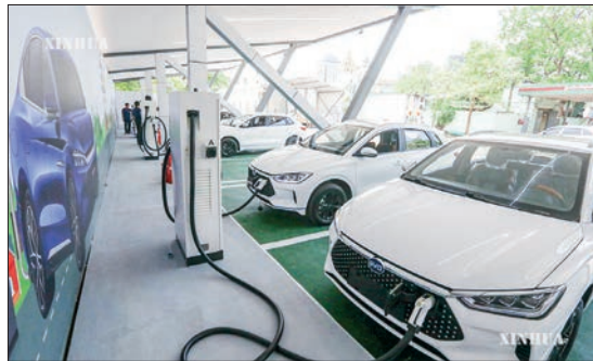
EV charging stations were opened at the front of Yangon Railway Station on 19 March 2023. PHOTO: XINHUA
