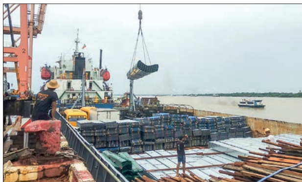
Construction materials being loaded onto ship at TMT port on 28 June.
