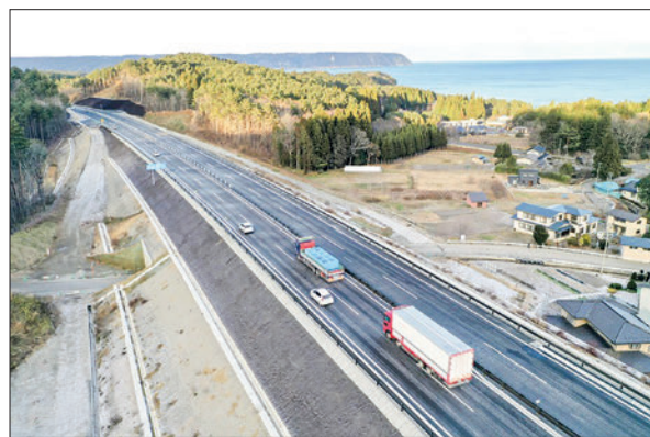
Photo taken 18 December 2021, from a drone shows a part of the Sanriku Coast Expressway in the Iwate Prefecture village of Noda, northeastern Japan. All parts of the 359-kilometre expressway between Sendai, Miyagi Prefecture, and Hachinohe, Aomori Prefecture, have opened in a state-run recovery project from the 2011 earthquake-tsunami disaster. PHOTO: KYODO
