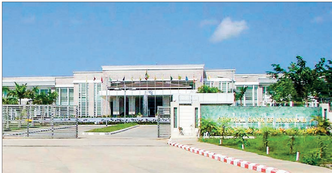
The office front view of the Central Bank of Myanmar.
