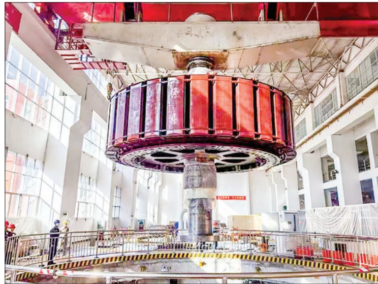
Engineers and technicians seen at successful lifting of the rotor of 2# generator set at Dapein (1) Hydropower Station in Myanmar.
