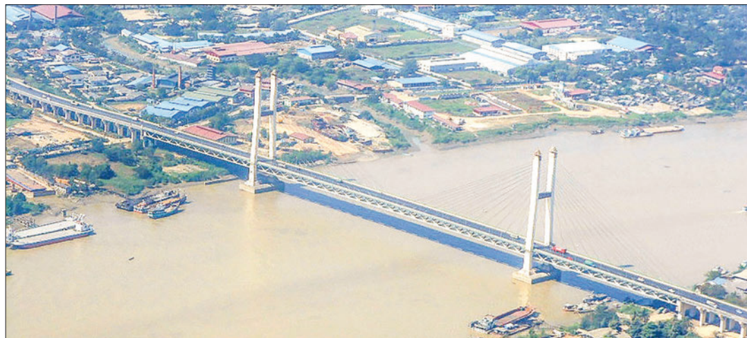
The photo depicts an area near Aung Zeya Bridge where an on-site wastewater treatment plant is to be built.
