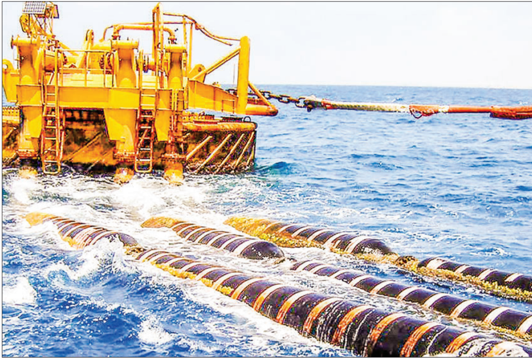
The photo shows the Myanmar-Singapore international underwater fibre cable transmission project.
