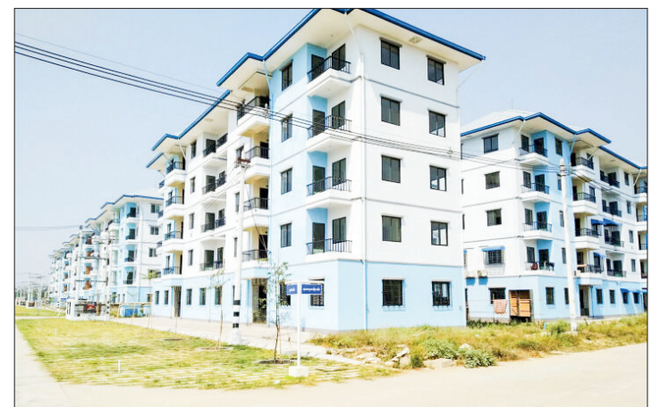
Photo shows completion of housings.
