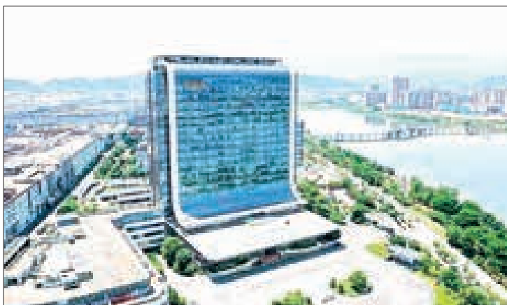
Aerial photo taken on 24 June 2022 shows the building of the Contemporary Amperex Technology Co., Ltd. (CATL), China's leading automotive lithium-ion battery maker, in Ningde, southeast China's Fujian Province. PHOTO: JI CHUNPENG/XINHUA
