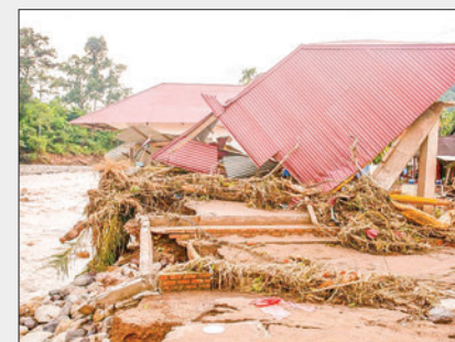
A house is left damaged after heavy rain at Pesisir Selatan Regency in West Sumatra, Indonesia, 10 March 2024. PHOTO: XINHUA
