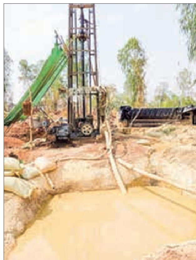
Mechanical digging a tubewell in the hot and dry zone.
