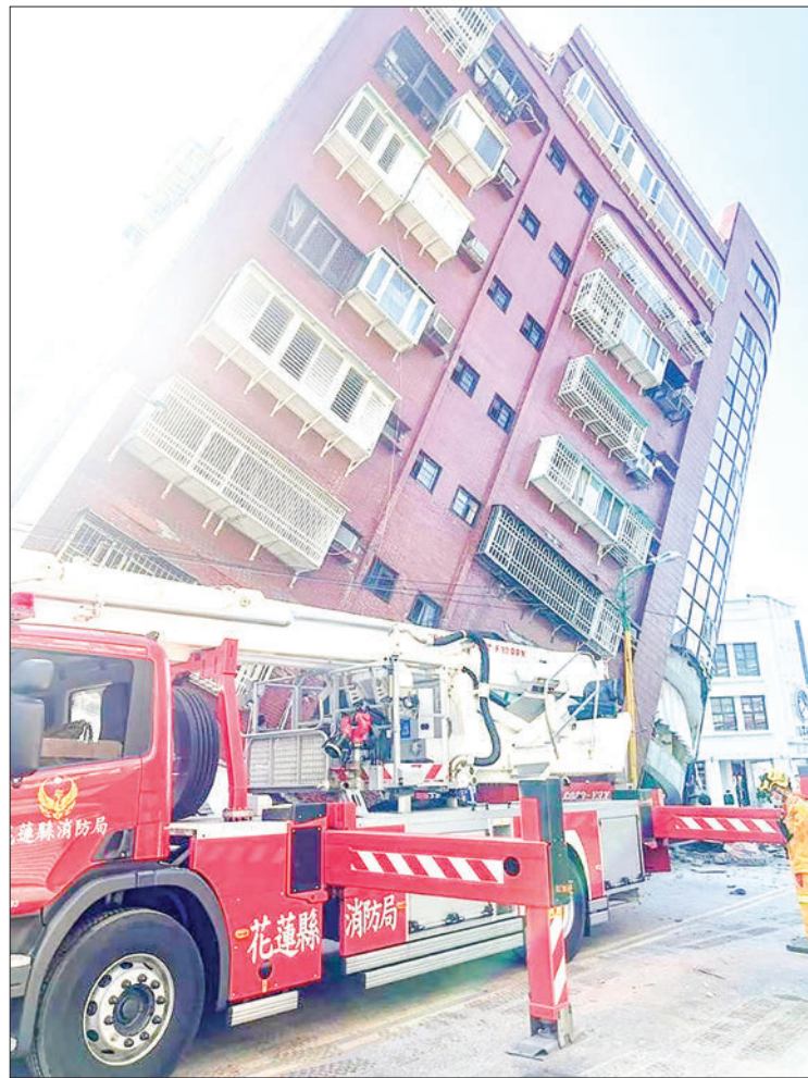
This photo taken on 3 April 2024 shows a damaged residential building in Hualien, southeast Chinese Taipei. PHOTO: XINHUA
