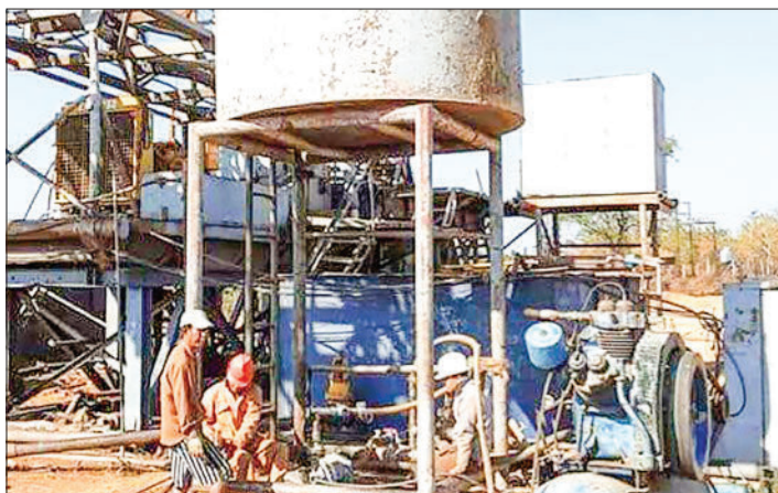
Petrochemical plant group (Thanbayakan).
