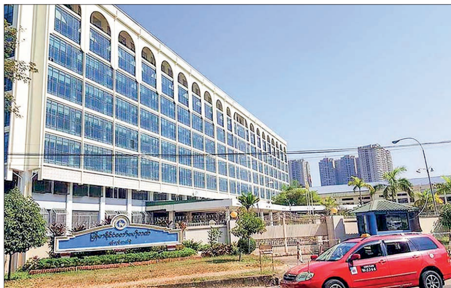
The office building of the Central Bank of Myanmar in Yangon.
