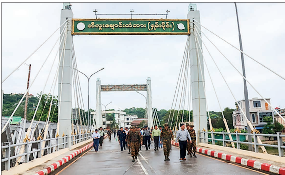
Kayah State Chief Minister U Zaw Myo Tin and Eastern Command Commander Maj-Gen Zaw Min Latt stroll along the Biluchaung Bridge (Shanpaing).
