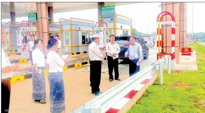
Deputy Minister U Win Pe seen inspecting the toll gate of the Thanlyin Bridge 3 yesterday.
