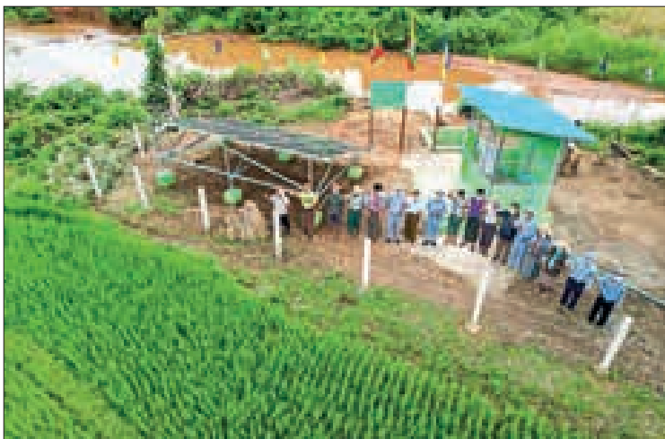
An aerial view of the agricultural water supply by solar system in Pindaya Township.
