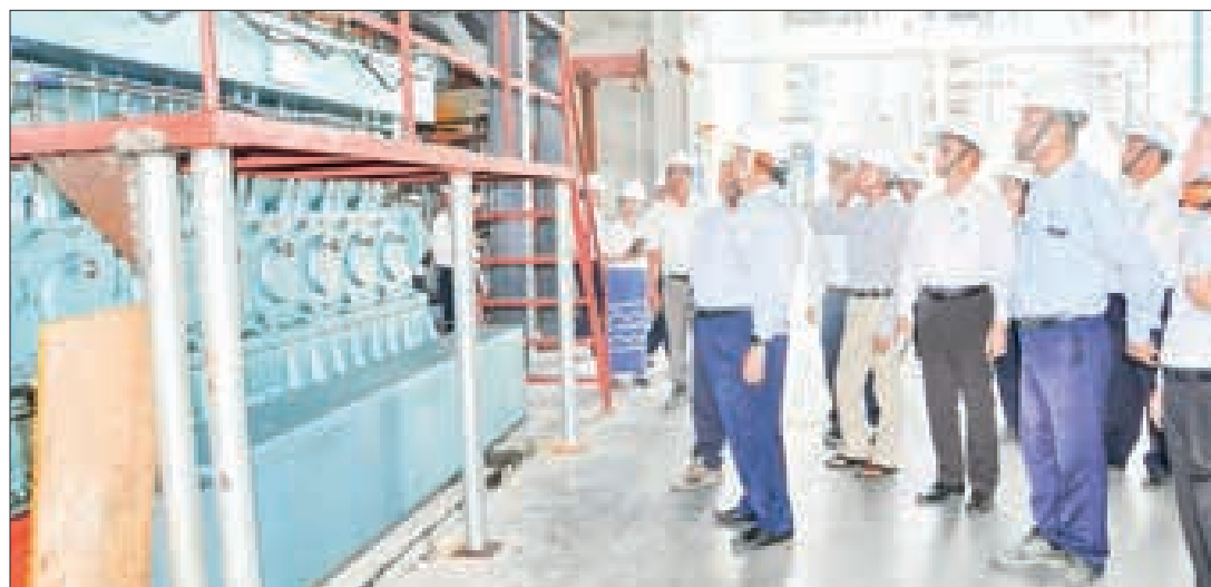
Union Minister for Industry Dr Charlie Than visits the construction site of the paddy husk gasification power plant in Ayeyawady Region yesterday.
