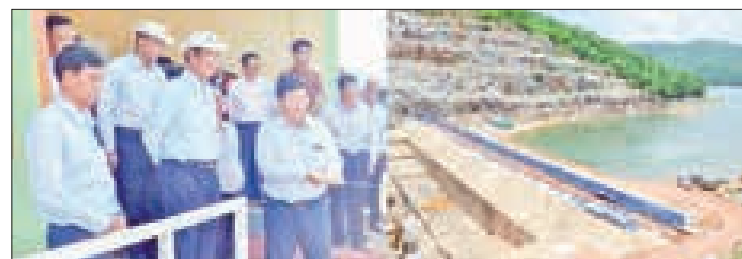
Union Minister for Electric Power U Nyan Tun observes the installation of the hydraulic elevator dam (HED) at the spillway of the hydroelectric power plant in Zeyathiri Township.
