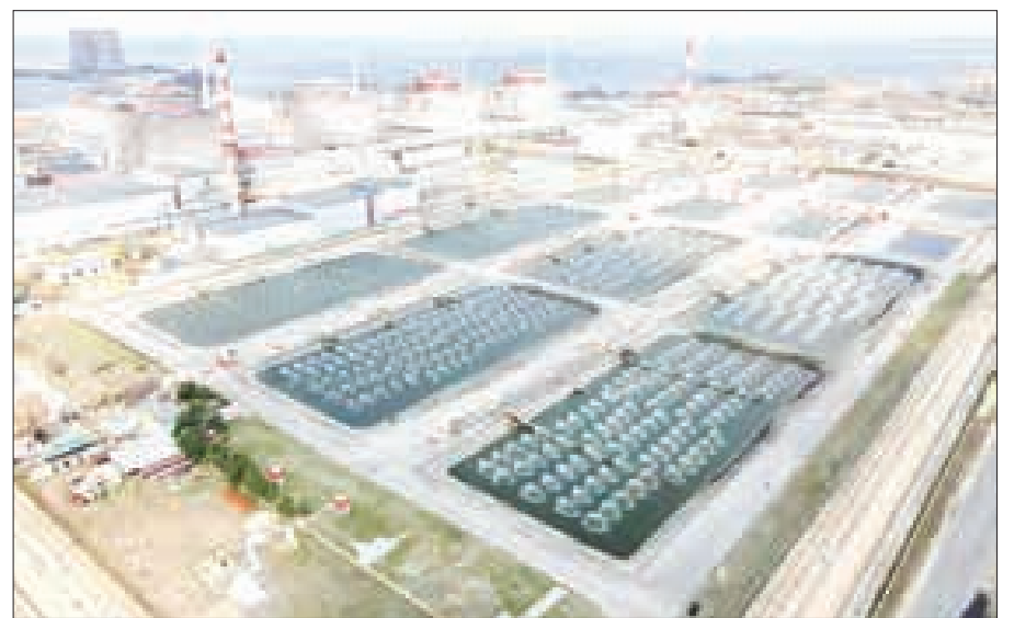
An aerial view shows the spray pounds at the Zaporozhye nuclear power plant. PHOTO: SPUTNIK
