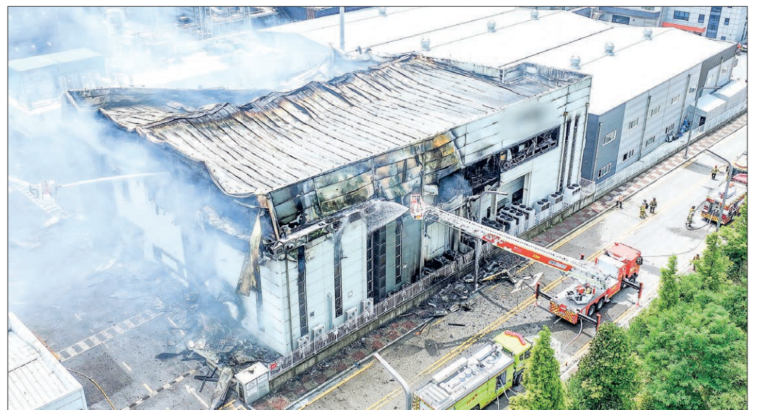
This photo shows an aerial view of firefighters working to extinguish a fire at a lithium battery factory in Hwaseong on 24 June 2024. PHOTO: YONHAP / AFP
