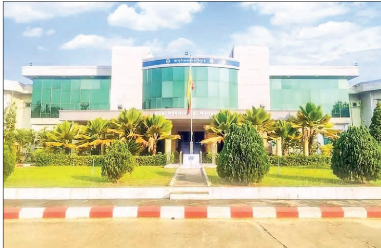
A front general view of the Ministry of Labour Office.
