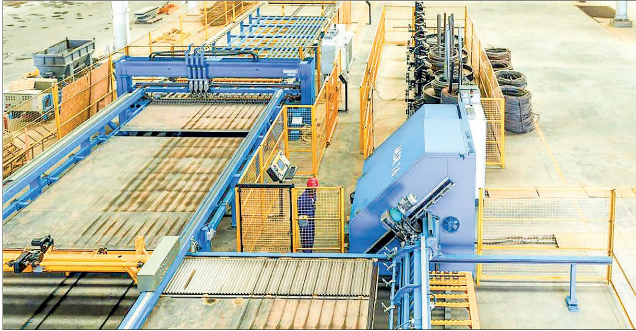
A staff member works at a workshop of China Wu Yi (Kenya) Precast Company Limited in the industrial town of Athi River, Kenya on 17 May 2024. PHOTO: XINHUA
