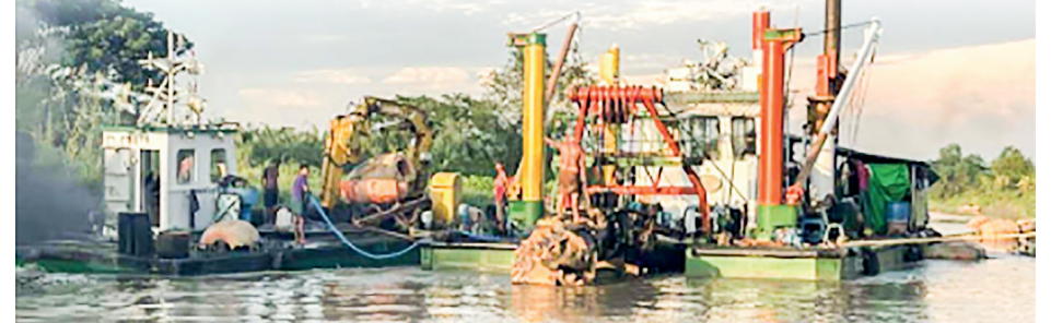
This picture captures re-excavation work of Ngamoeyeik Creek.
